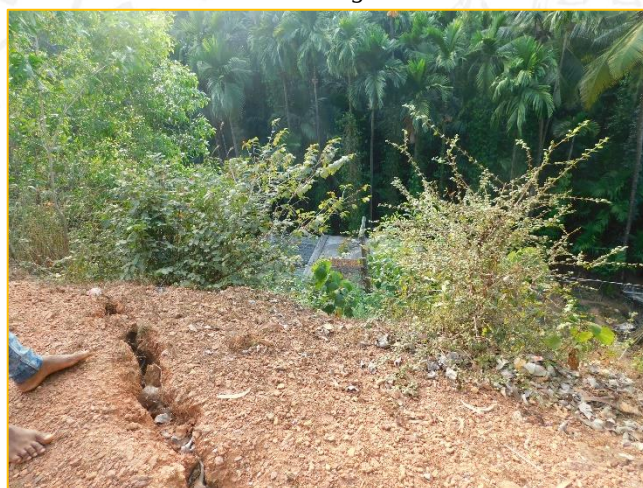
Photo 3. 3b, Slope cut failure near Kodani village- Ground cracks Lat: 14° 1'3 53.24" Long: 74 34' 1.88"
