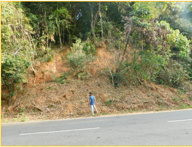
Photo 3. 4a, Soil slide along NH-206 Lat: 14°13' 44.85 "Long: 74° 48' 58.51"
