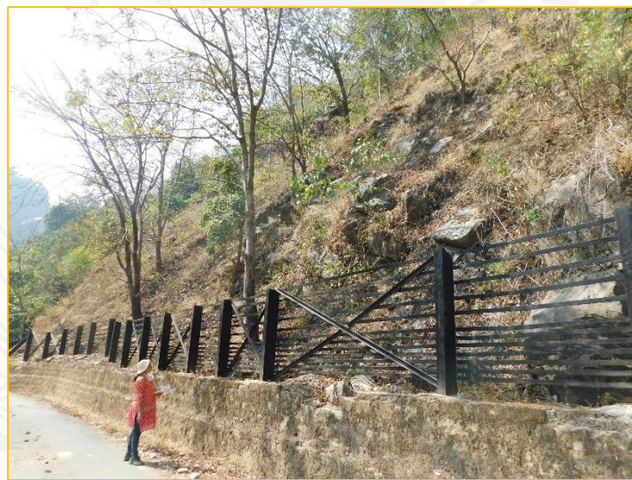
Photo 3. 5, Towards Mahatma Gandhi power station- Iron crib wall to prevent the rock slides.
