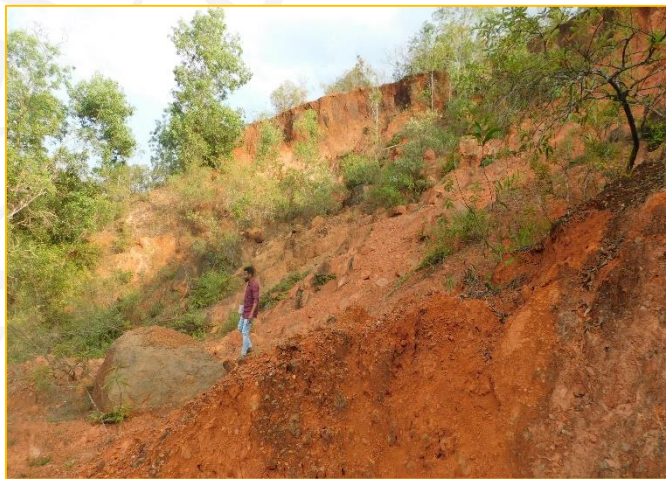
Photo 4.k, Loose slide debris
